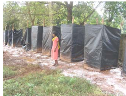
Temporary Toilets constructed by JRP
